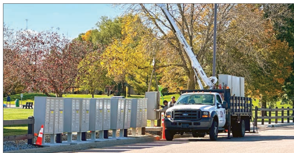
CONSTRUCTION CREWS began installation of the Post Office boxes behind the Becker Community Center. Keys for the boxes were also distributed and boxes should have been ready to use by earlier this week. (Submitted Photo by Scott Boerner).
