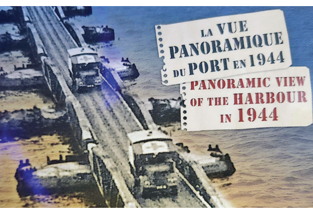
MULLBERRIES BRIDGES BUILT IN THE WEEKS BEFORE NORMANDY (left photo) locked together and were 280' x 50' wide x 65' deep metal segments bridges that went far into the water and then to shore to transport nearly 100% of landing craft, troops and materials up the beach. (Submitted Photo).
